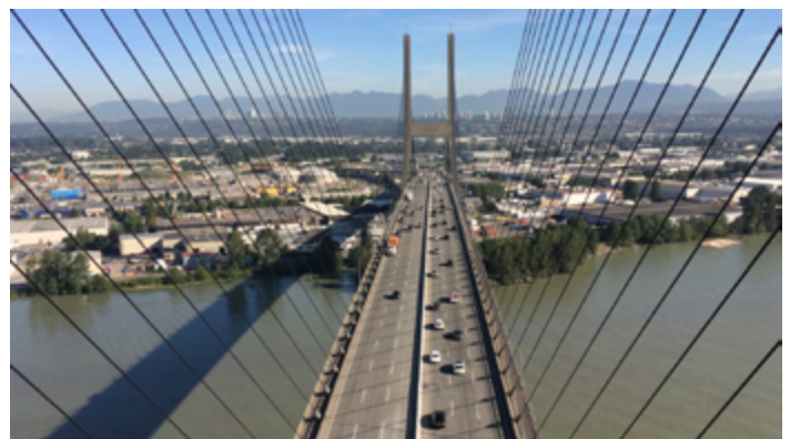
The Alex Fraser Bridge
